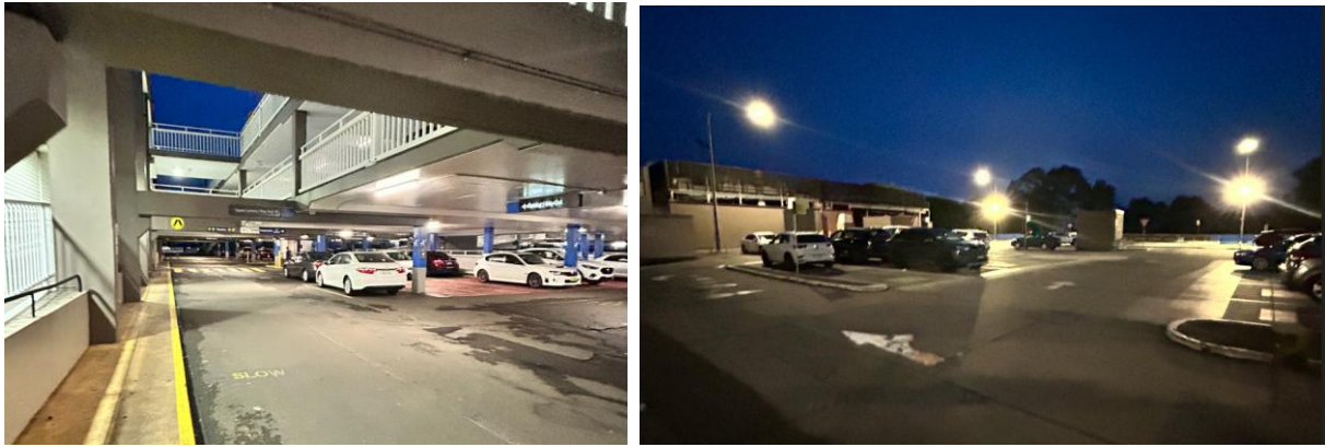
Parking area- surveillance, signage, access from the centre and lighting (night time)
