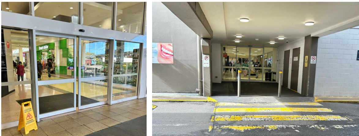
Other entrances to the site: to the left is the secondary entrance via Roselands Avenue (next to the main entry), and to the right is the western entrance from the carparking
